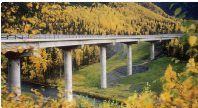
Figure 1-1 Often simply paying attention to proportions and details can result in an attractive bridge with no increase in cost. Canyon Creek Bridge, Anchorage, Alaska.
